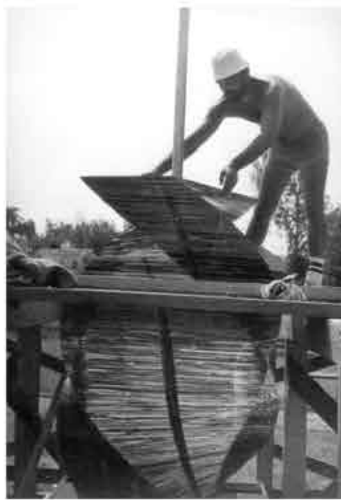
THE METHOD OF BUILDING FLAKY GLASS SCULPTURE (AFTER HAVING THE PRE-FABRICATED ELEMENTS)
